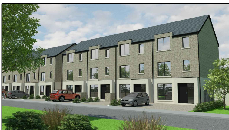
Townhouses (Terrace 02) - Character Area 1 See site plan (dwg no. 20068/P/003) for material locations
